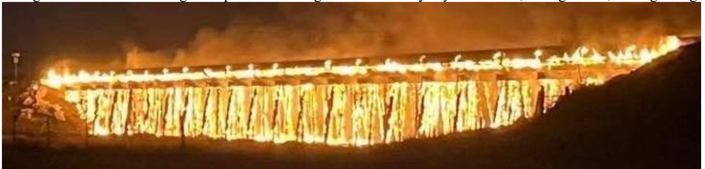
A still from a video showing the BNSF trestle outside of Canyon, TX ablaze. (Photo by Amarillo Fire Dept.)
