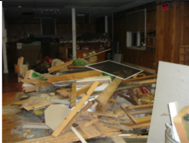
Tinplate layout demolition before move to Front Room – 2004
