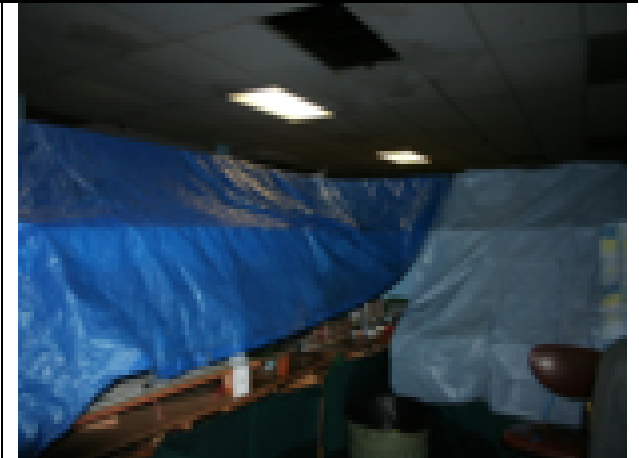
HO layout covered from storm damage 2011
