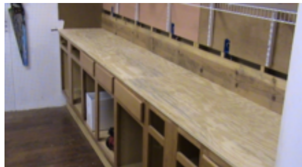
Finished storage unit
